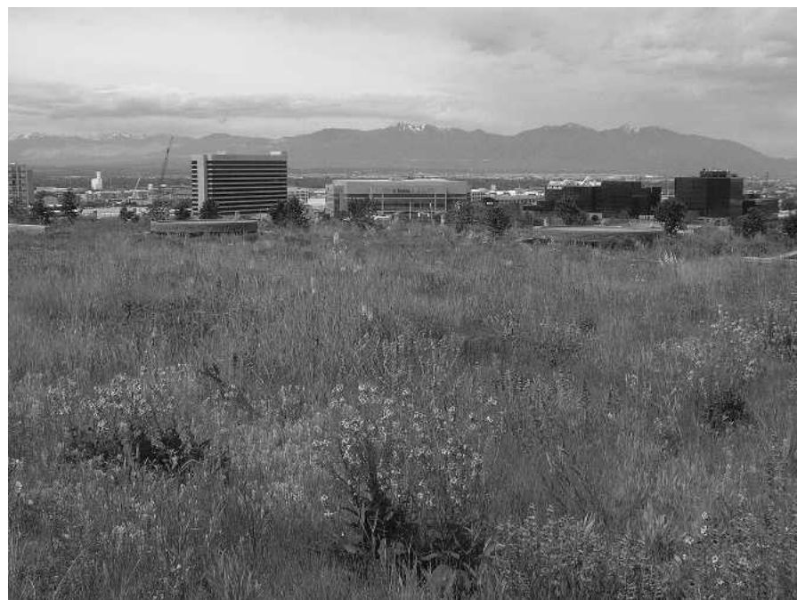
Fig. 4. An extensive green roof native plant community on the convention center of the Church of Jesus Christ of Latter-day Saints in Salt Lake City, Utah.
