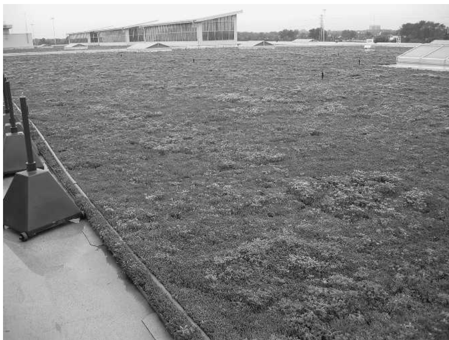
Fig. 2. Portion of a 10.4-acre extensive green roof on an assembly plant at Ford Motor Company in Dearborn, Mich. Plant material consists of 13 species and cultivars of Sedum .
