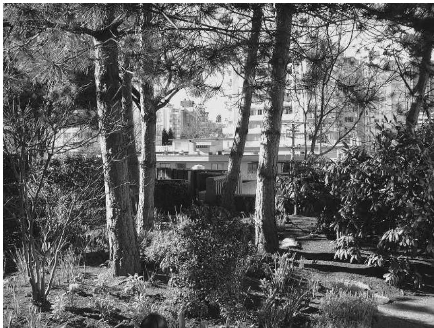
Fig. 1. An intensive green roof on the Coast Plaza Hotel in Vancouver, British Columbia.
